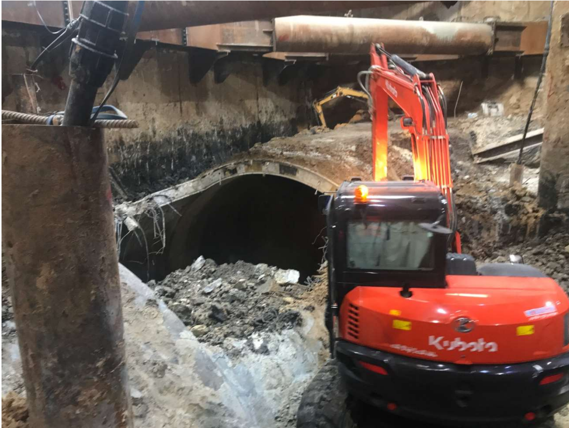
Figure 5– Demolishing one of the tunnels at Shaul Hamelech Station
